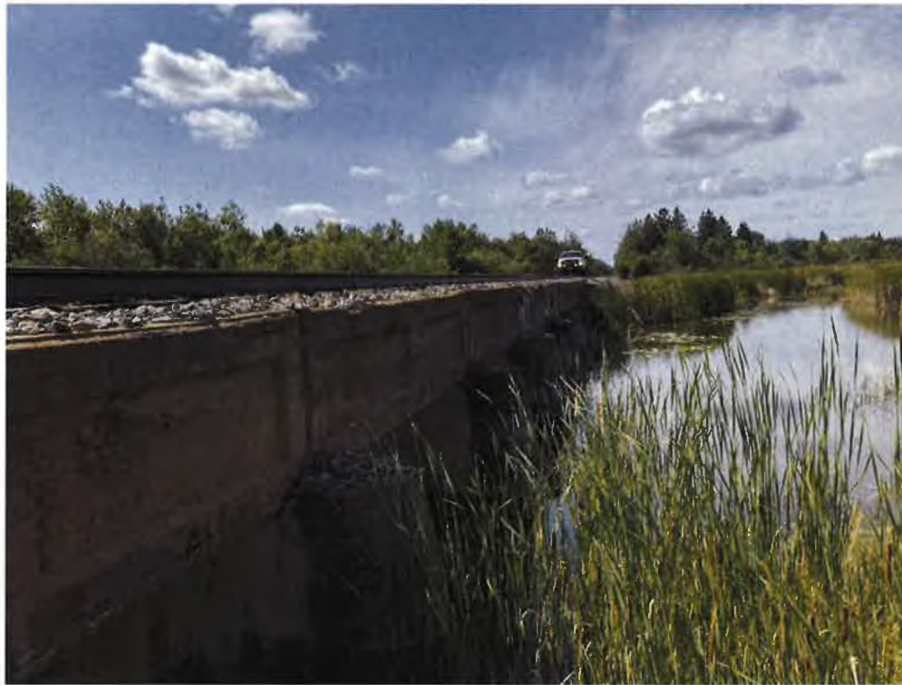
Upstream Side Looking Southwest
